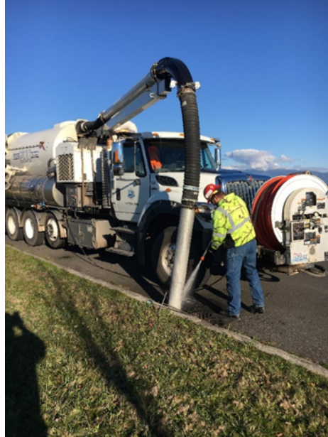
Figure 5-1. Skagit County's vacuum truck used to clean a catch basin.
